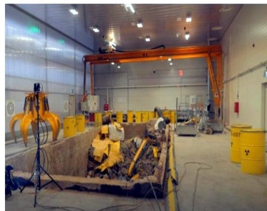
Figure 7. Operation inside the primary containment during waste retrieval
