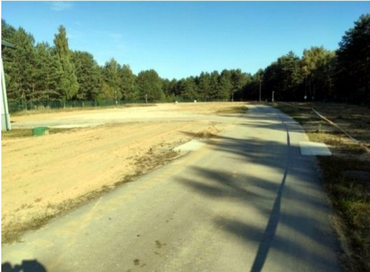
Figure 16. Site condition after decommissioning works (cropped from the final report appendix).
