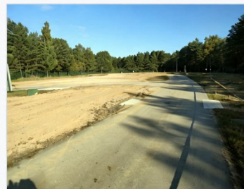
After decommissioning / site remediated
