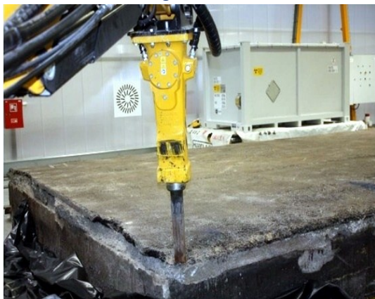
Figure 8. Cold testing / start of remote demolition of the upper part of vault “r1”
