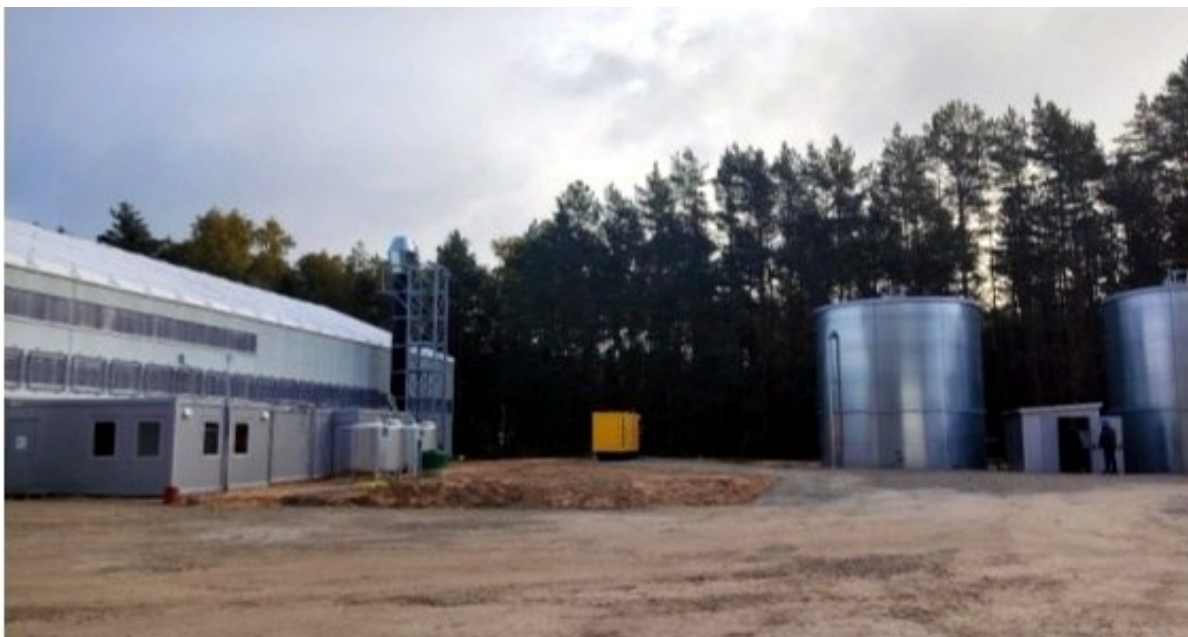
Figure 14. Temporary infrastructure installed to support safe waste retrieval and decommissioning operations
