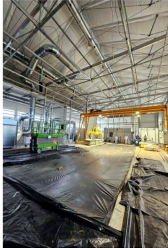
Figure 10. Caisson / temporary structure context supporting safe retrieval and dismantling
