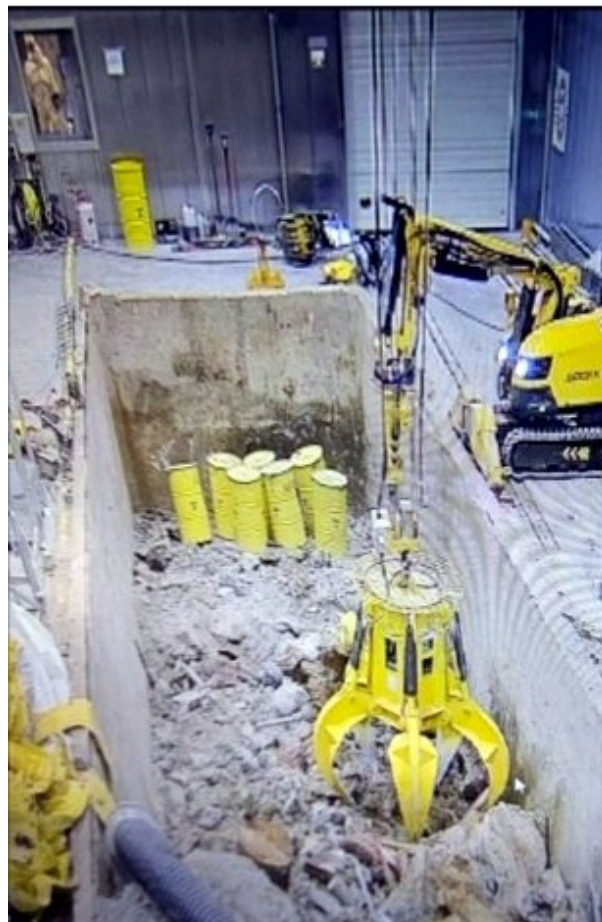
Figure 11. Remote handling during retrieval operations
